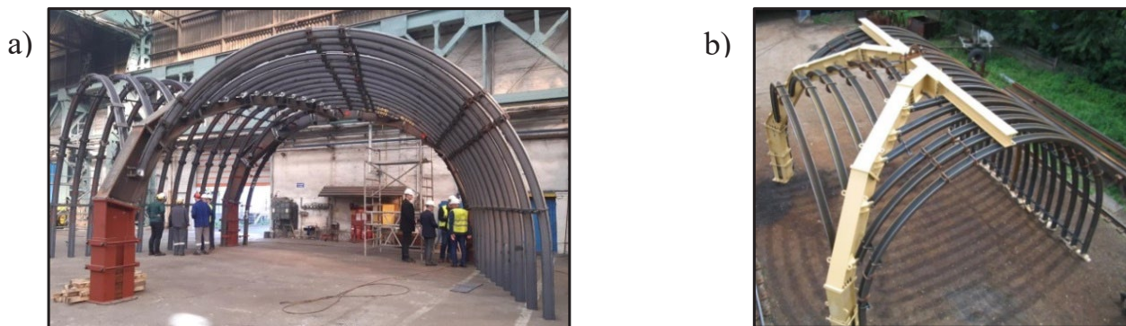
Figure 3: Examples of portal support implementation for three-way junctions: (a) at an acute angle and (b) at a right angle (Rotkegel, 2015).
