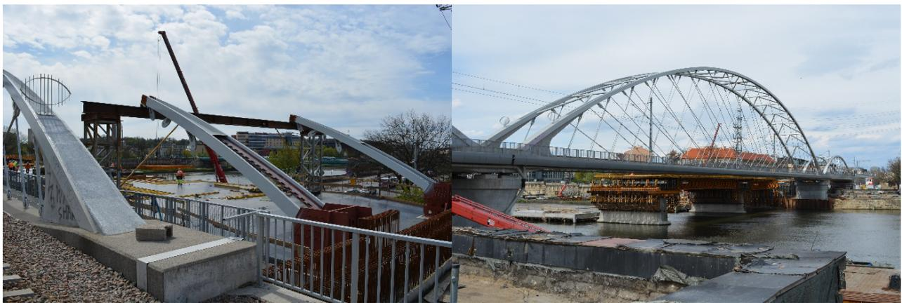
Figure 10: Photos of network arch bridge over Vistula River in Cracow (own source).
