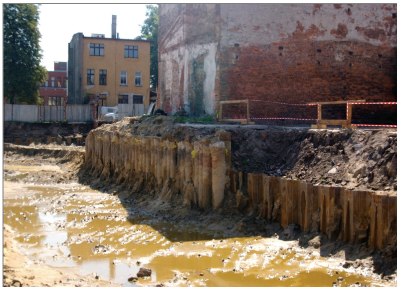
Fig. 2. Pile wall view
