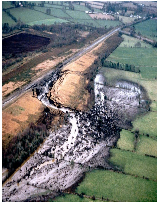
Fig. 3. Slide on Grand Canal embankment (PIGOTT et al. 1992)
